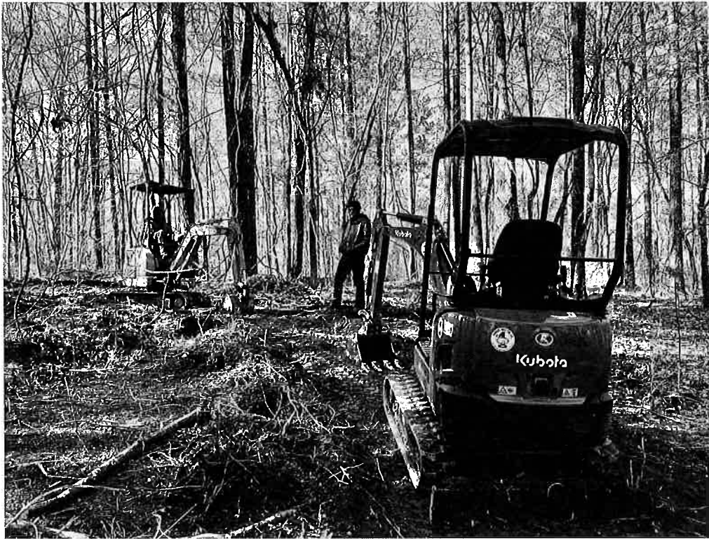
Mountain bike trail building at Chattahoochee Bend State Park
